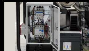
The earth leakage protection option will protect people against electrical shock in the event of indirect contact.
